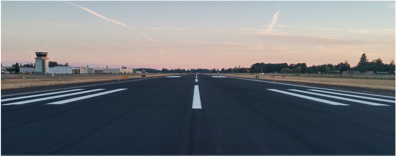
Runway 17 Looking South – Source: Century West Engineering
